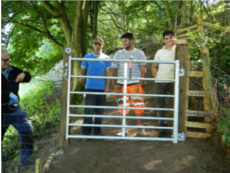
Bridleway repair and maintenance
