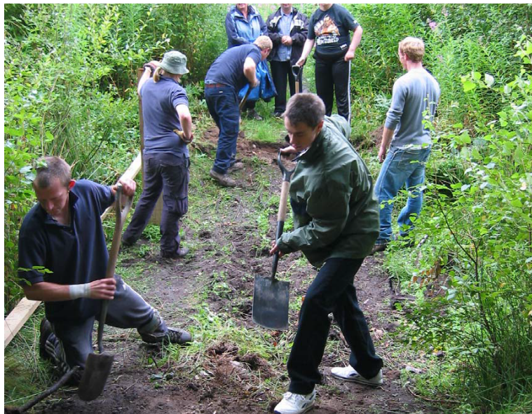
Shropshire Outdoors Project – Volunteers working alongside our Access Maintenance Team
